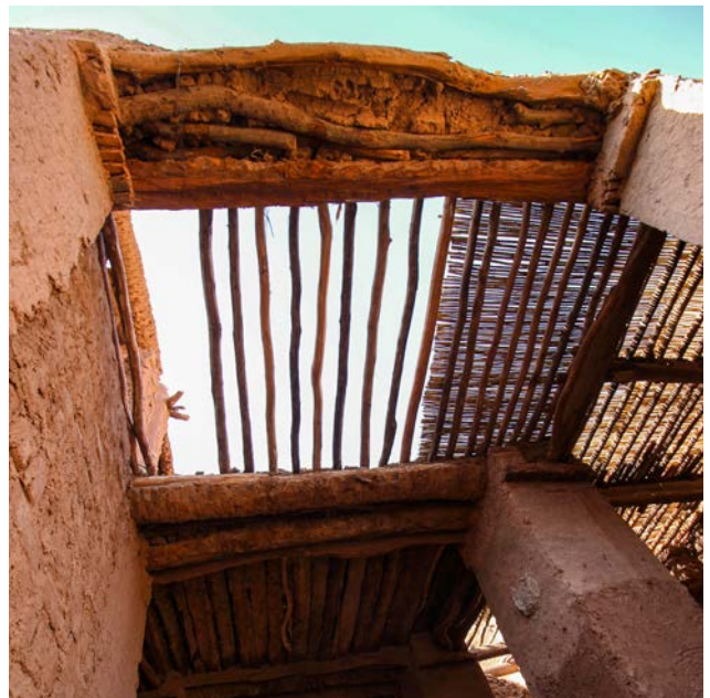
Roof construction with tamarisk branches and reed mats
