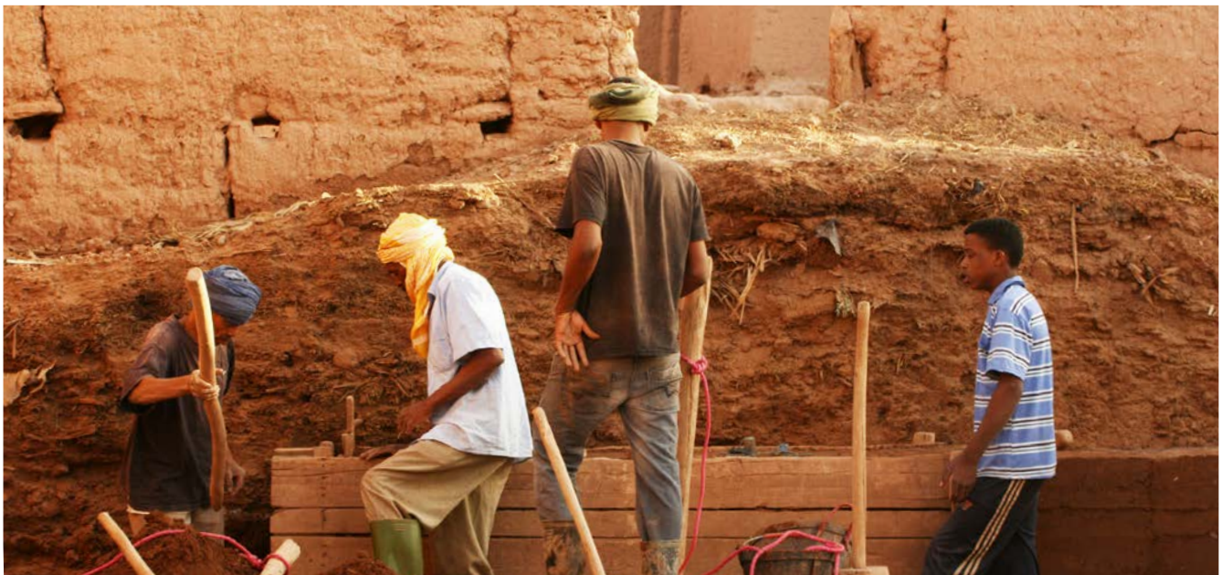
Construction of a rammed earth wall
