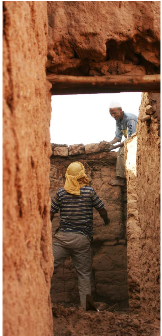
Master builder and assistant rebuilding a rammed earth wall
