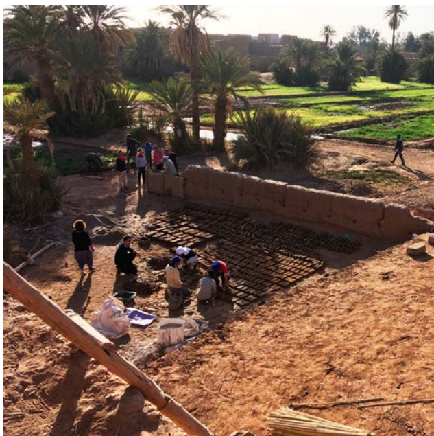
Mud bricks making and rammed earth wall construction
