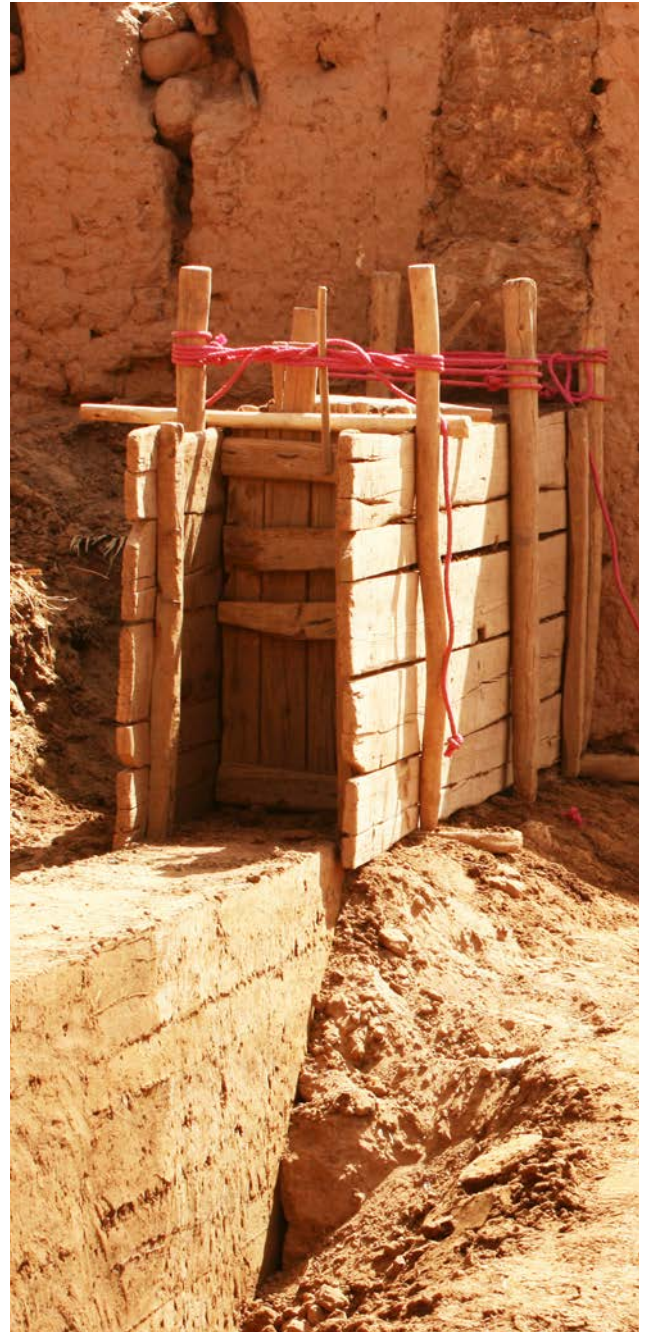
Rammed earth wall and wooden formwork
