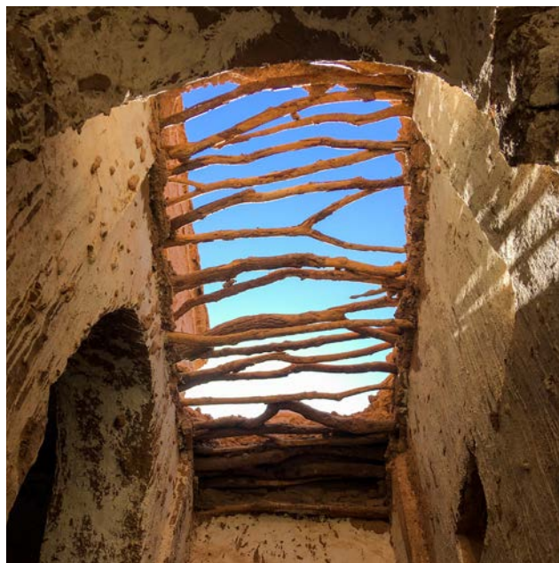
Timber roof of the marabout before restoration
